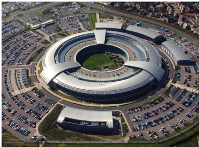
The United Kingdom's Government Communications Headquarters (GCHQ) was forced to reveal its policy on mass surveillance. Creative Commons, Flickr / UK Ministry of Defence
